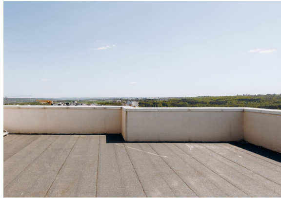
Example of parapet cap
