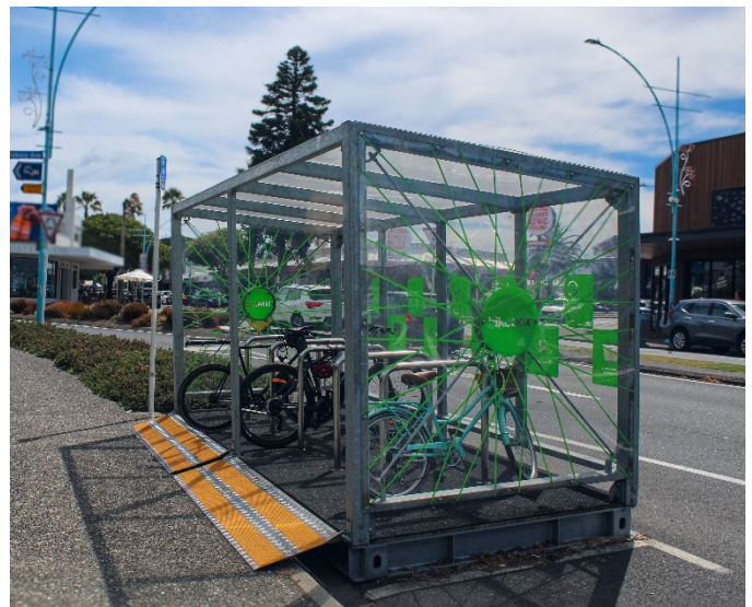
Example of weather-protected bicycle parking
