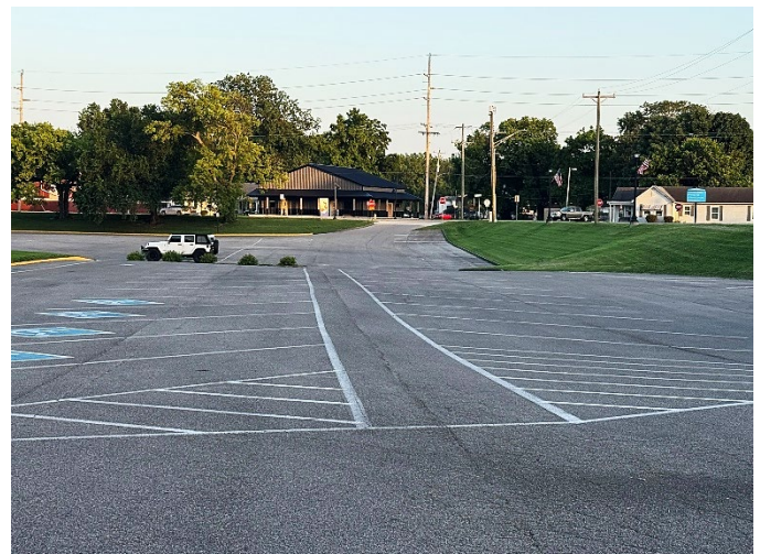
Example of striped pedestrian connection through a parking lot
